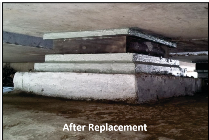
Photo 2 : Photograph of a typical bearing before and after replacement.
