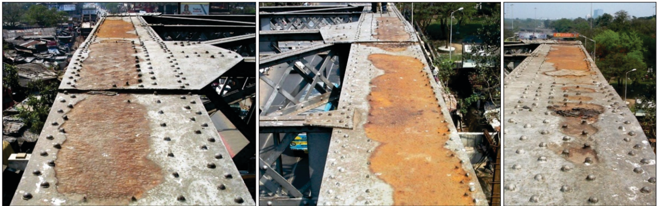
Fig. 12 : Photo showing extent of top-chord corrosion in the bridge
