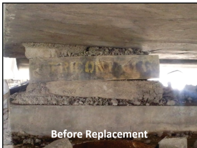
Photo 2 : Photograph of a typical bearing before and after replacement.
