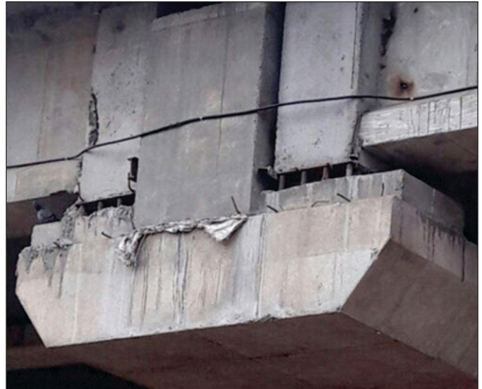
Photo 1 : Hanging Sleeves from Bearing top plate
