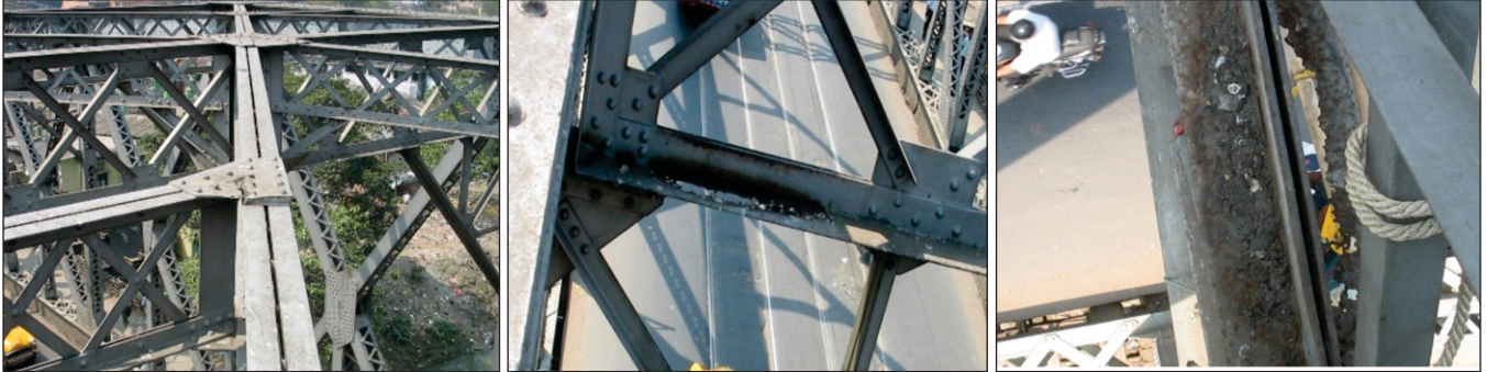
Fig. 13 : Photo showing extent corrosion in the Lateral Bracings & Portal Joints
