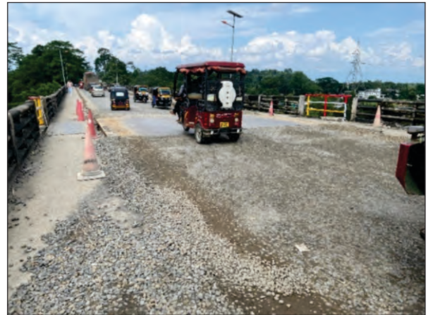
Photo 10 : Bridging Span created at middle of P1-P2 to bypass Suspended Span
