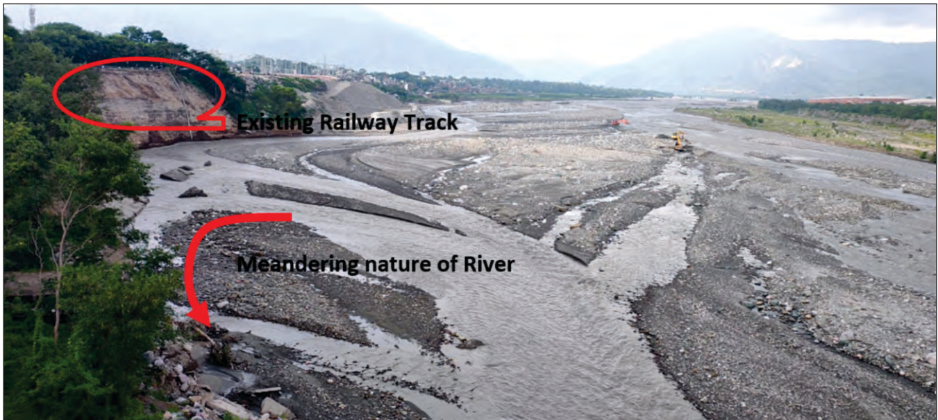
Fig. 2: Meandering nature of River causing Embankment Erosion on Up Stream Side on Outer Embankment
