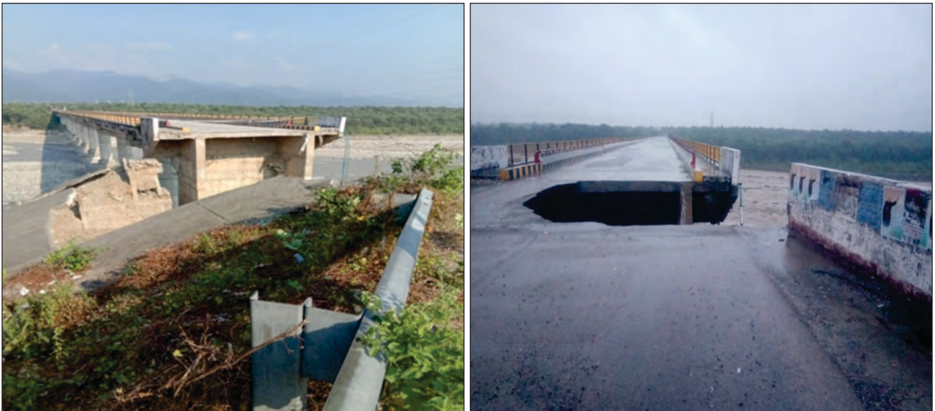
Fig. 1: Approach Road behind Abutment A1
