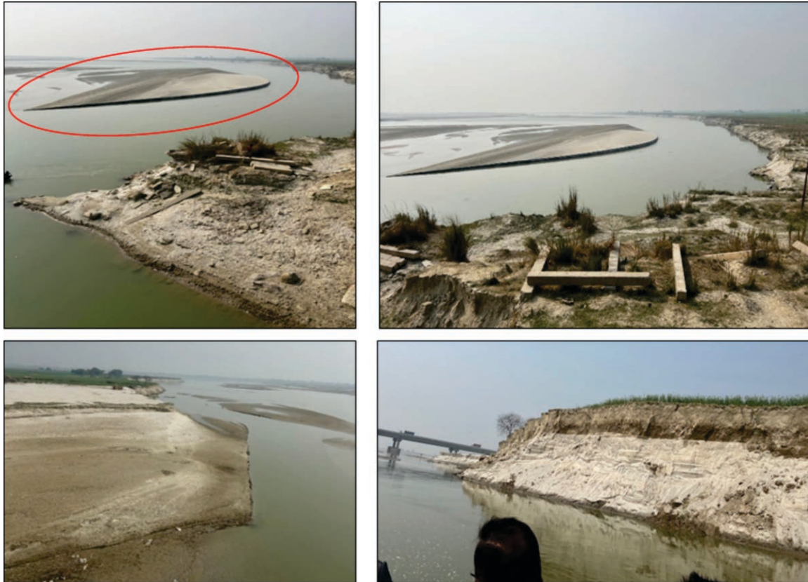
Fig. 3 : Showing Shifting tendency of river towards Left Bank side during previous years (Alarming situation w.r.to shifting during March.2024 to Dec.2024)
