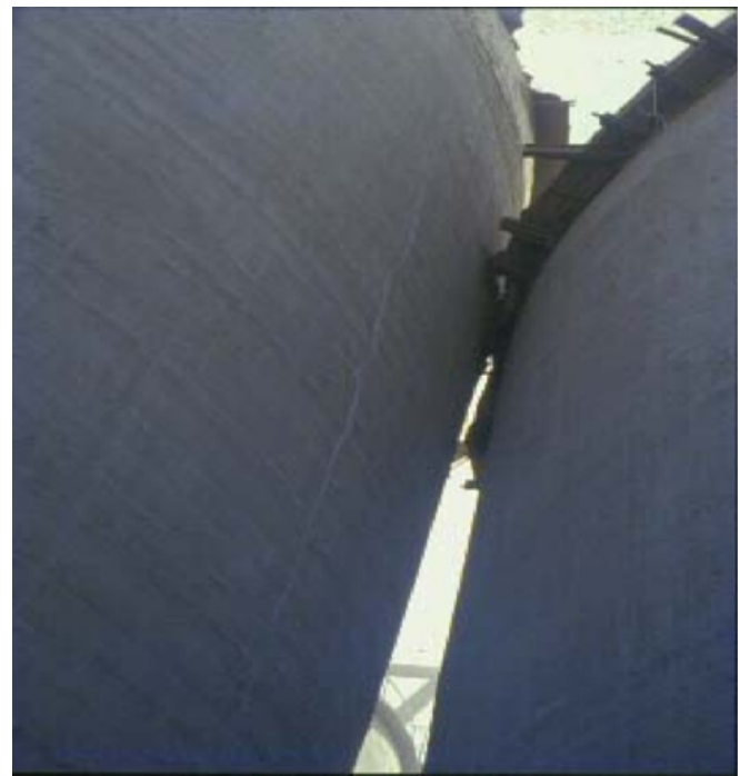
Fig 4 : Tilted Silo
