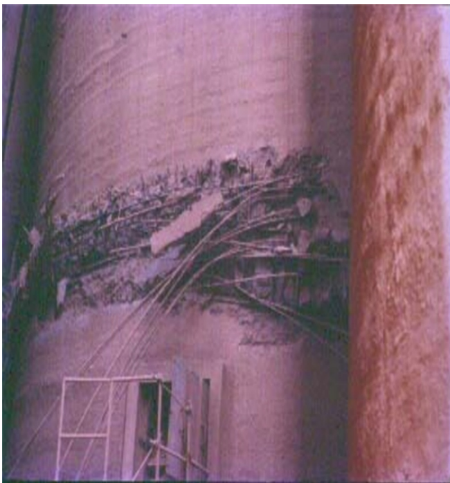
Fig 3 : Crushed Concrete
