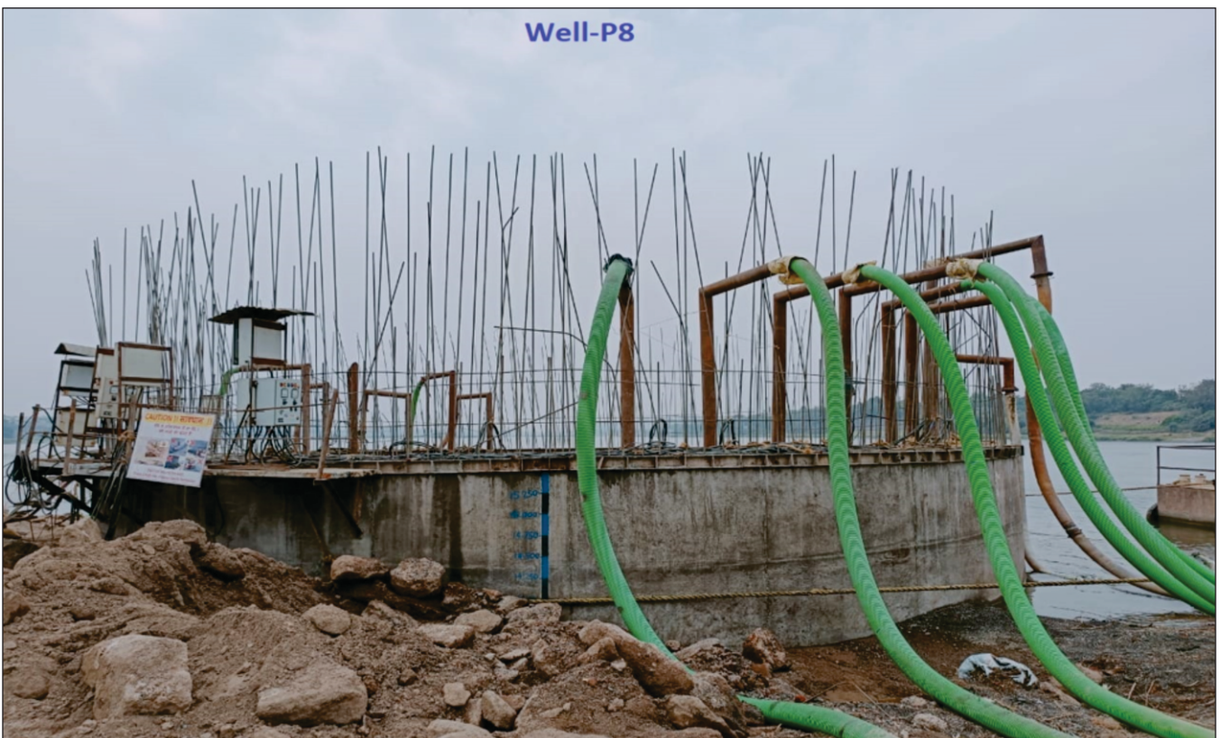
Fig. 3 : View of the Well from top showing arrangement of pumping to dewater
