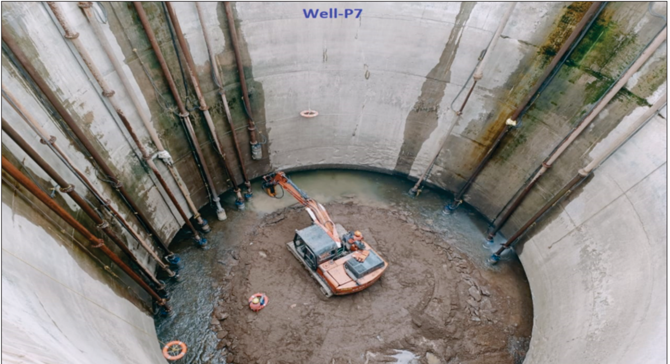
Fig. 2 : View of the dredge hole for well P7 where attempt is being made to cut thru' rock. Pumping-out of water is simultaneously done to ensure dry condition for ease of working
