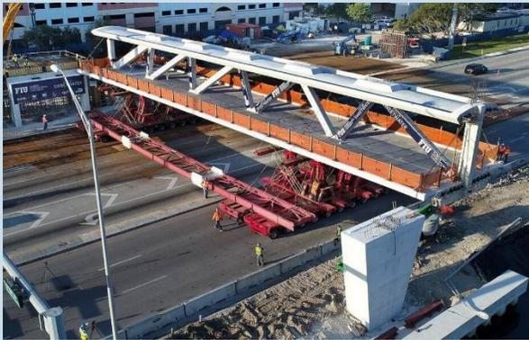
Fig.4 Photograph of the span being positioned over support.
