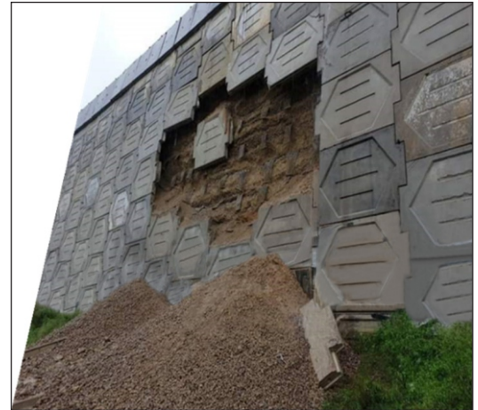
Fig. 3 : Failure of MSE Wall due to connection
