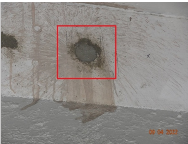
Fig. 3 : Concrete Core cut sample has been taken from basement beam.
