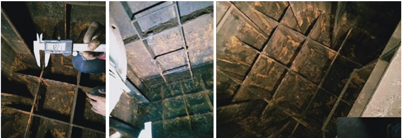
Fig. 2 : View of the corroded steel pier box from inside
