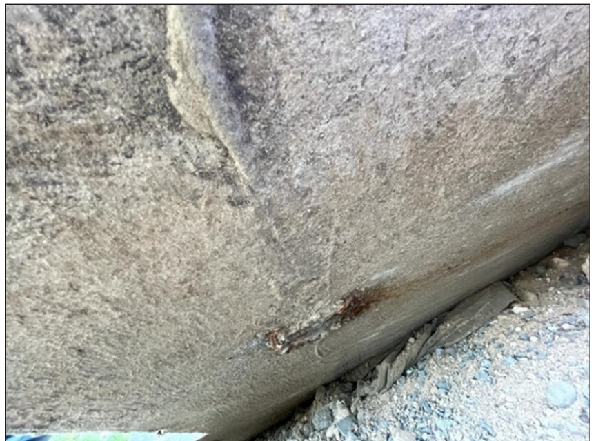
Fig. 2 : Connection failure at closing wall and collapse of panel
