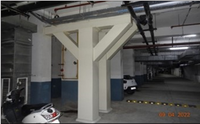
Fig. 1 : Some basement beams are supported by fabricated steel columns.
