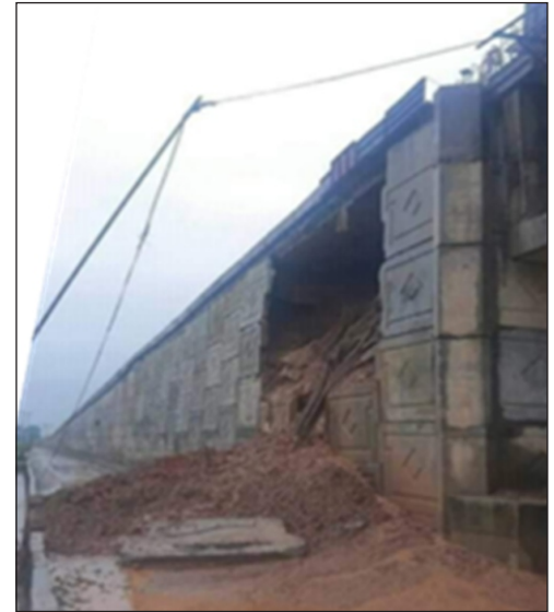
Fig. 1 : Failure of MSE Wall for Case Study
