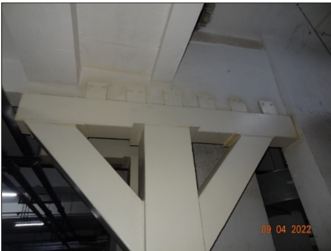
Fig. 2 : Side view of the steel column supporting the basement beam.
