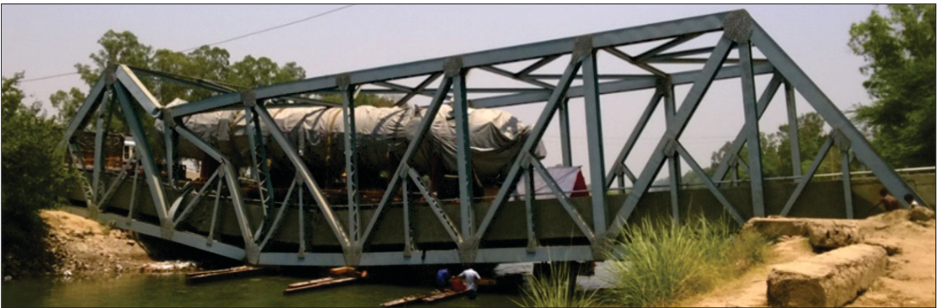
Fig. 1 : View of the Collapsed Bridge Over Canal
