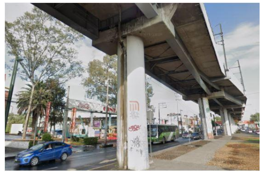
Fig. 2 The Overpass before the accident (2019 Photo) (Source: Ref. 6)
