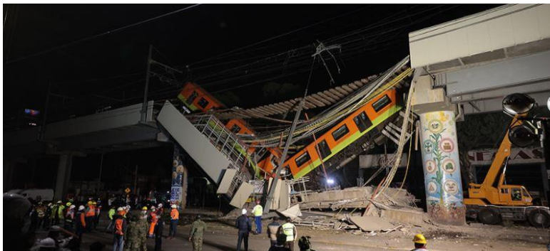
Fig. 1 Collapsed girder supporting an overpass carrying Line 12 of the Mexico City Metro (Credit: Reuters Photo)
